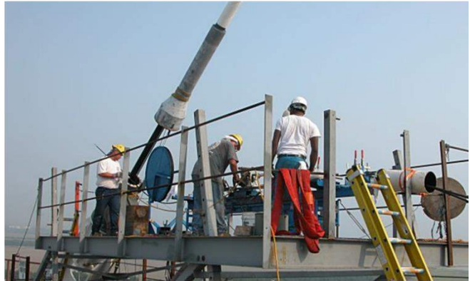
Pull –In and Stress Strands, one after the other
