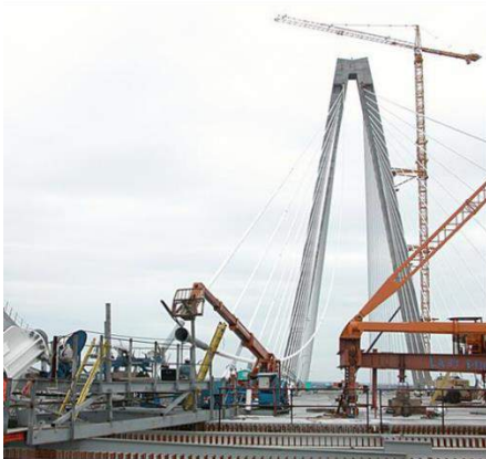
HDPE Duct gets inserted
